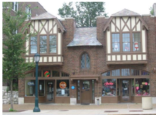
AFTER: Siding has been removed; Transoms are restored to original glazing pattern; Storefronts are appropriate wood construction; Trim and panel details have been restored at facade.
